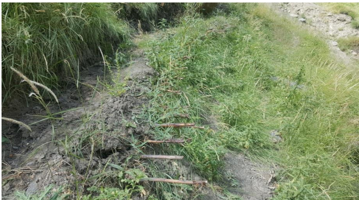
Figure 3: Bioengineering in Bhar Valley Nagar for Slope stabilization (PMCC, 2019)
